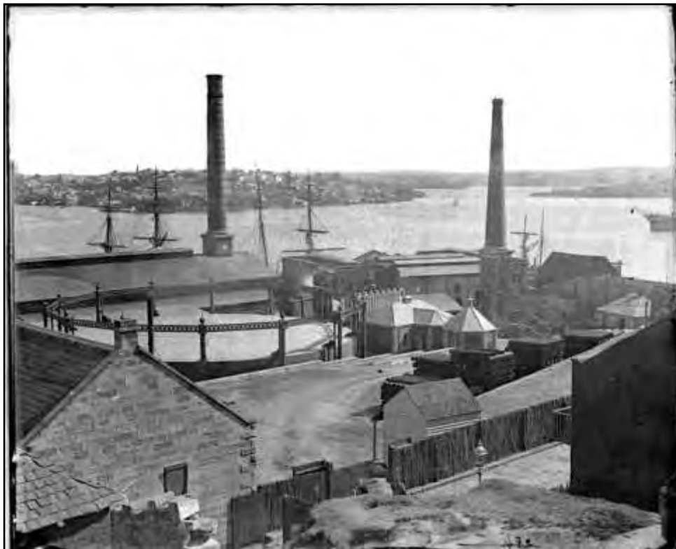
Australian Gaslight Company, Jenkins Street, Sydney (Millers Point) showing gasholder in middle ground – from State Library of NSW
