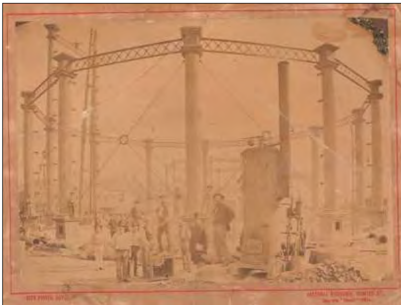
C. Lewis Construction Team Building Largest Gas Holder in Haymarket First Light: 150 Years of Gas
