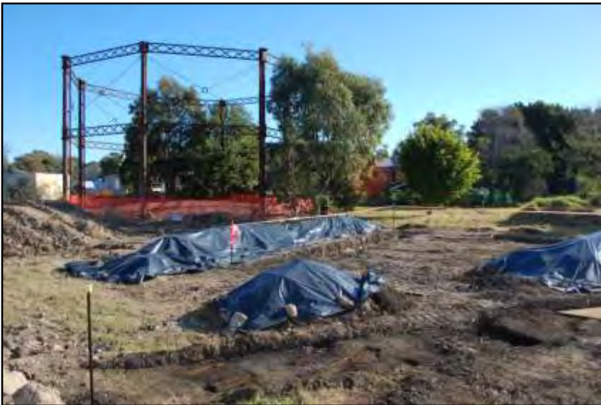
Site excavation photo with southern gasholder in background from 2010 excavation.
