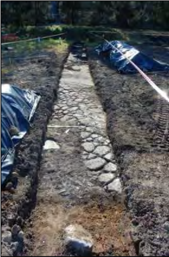
Trench 3 from 2010 excavation exposed concrete paving, cracked and revealing stress lines from wall or heavy machinery.
