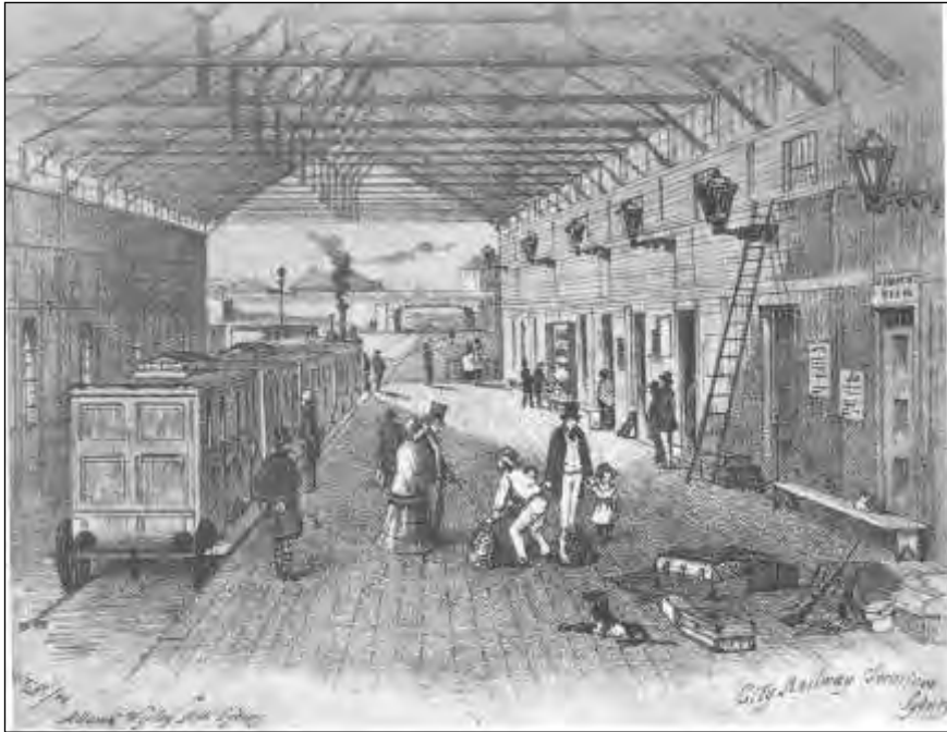
“City Railway Terminus Sydney”, showing gas lamp lighting First Light: 150 Years of Gas
