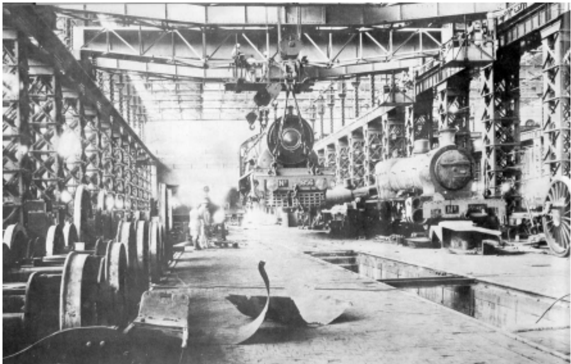
Figure 3.142: The erecting shop of the Locomotive Works at Moghulpura. This photograph is undated but was taken before Independence in 1947, when the works belonged to the North Western Railway. They became part of the Pakistan Western Railway on formation of Pakistan. Source: 'Encyclopedia of Railways' p 78.
