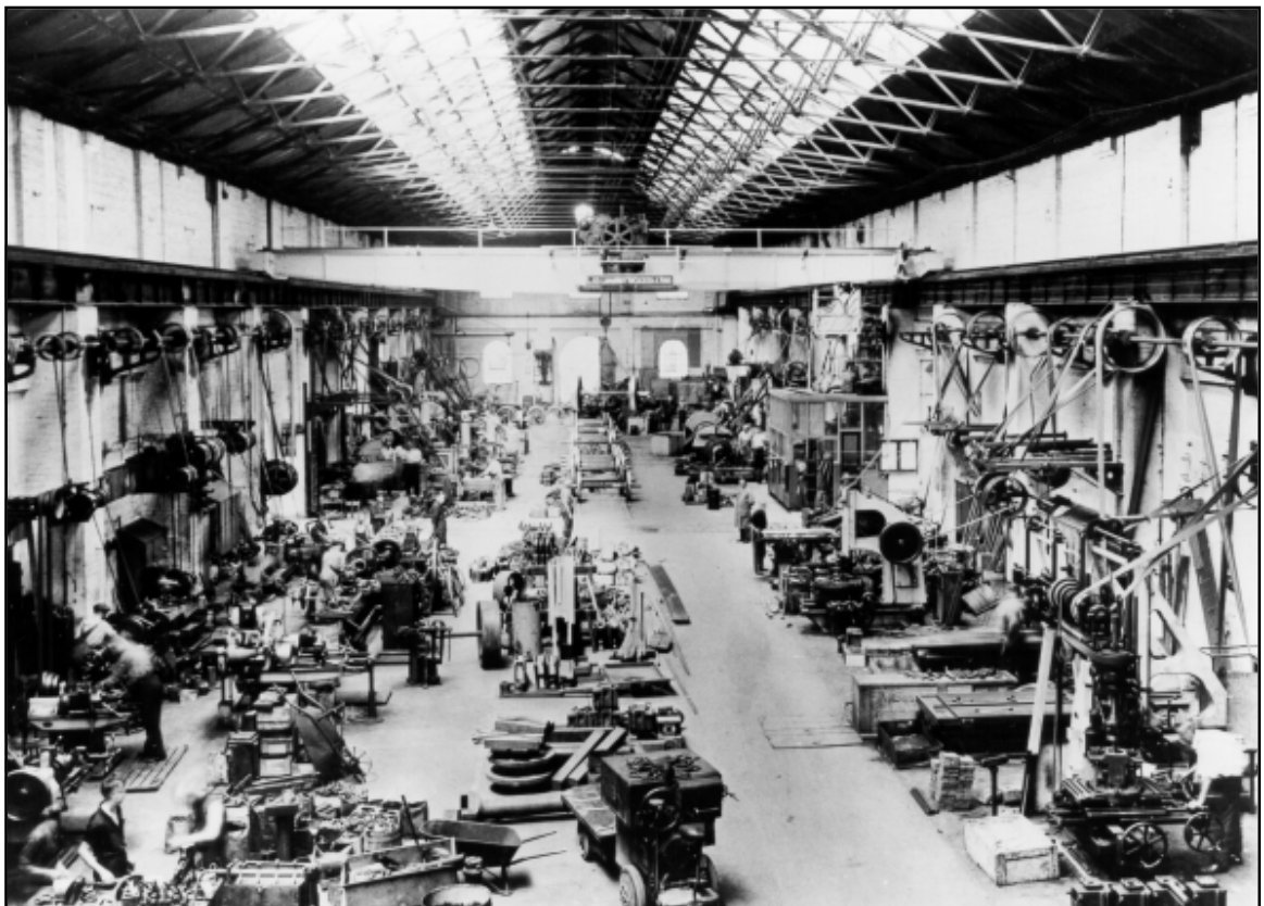
Figure 2.0: Interior of the Fitting and Turning (Machine) Shop, Bay 21, Carriage and Wagon Workshops, undated. This shows the overhead travelling crane, line shafting and counter shafts and belt drives to the machinery along each side of the bay. The central area contains stored raw materials and finished items and the rear sets of wheels. There is a timber office, probably for a foreman, part way down the right hand side of the bay. Natural day light is provided by the skylights and no artificial supplementary lighting is evident. This photograph is looking south from the mezzanine which was over the steam, later gas, engine which provided power. Source: SRAO
