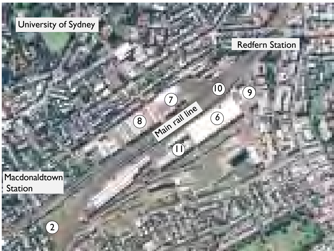
Figure 2.3: 2002 aerial photograph of the Eveleigh Railway Workshops complex showing items referred to in this report. Some items in the key have been demolished and are not shown.
