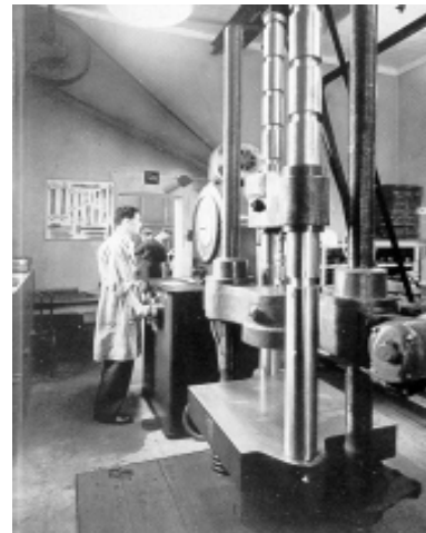
Figure 3.49: The Tensile Testing Machine in the Engineering Division of the Laboratories in 1955. The building in which this photograph was taken is now Scientific Services Building No. 1. Source: 'The Railways of New South Wales 1855-1955', p. 243.
