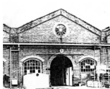
Figure 3.168: Newport Railway Workshops, Melbourne. The composition of the building is less formal than Eveleigh. At Newport the gable is expressed as a pediment and the windows are semicircular arches. Generally the buildings are similar with face brickwork divided into bays and forming a parapet, polychrome work around openings, the bulls eye window and the central opening, Doring, Newport.
