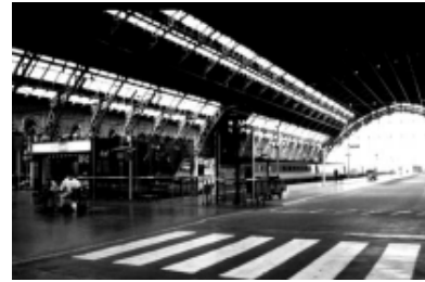
Figure 3.137: Interior of St. Pancras Station, London, a spacious hall made possible by the use of new iron technology. Source: Kate Mountstephens, 1998.
