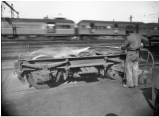
Figure 3.69: Two views of bogies being cleaned at the Eveleigh Carriage and Wagon Workshops. The view on the left is taken adjacent to the main lines, probably on the apron outside the Paint Shop. The view on the right is on the northern side of the Carriage Workshops near the Blacksmiths' Shed. Undated. Source: SRAO
