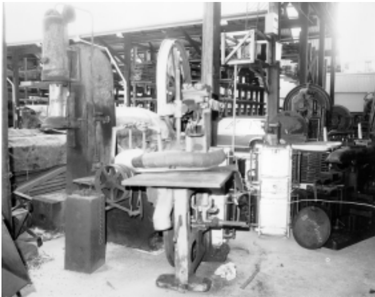
Figure 3.96: Carriage workshops 1989. The pedestal hydraulic press and belt driven bandsaw await removal to another site or scrapping.
