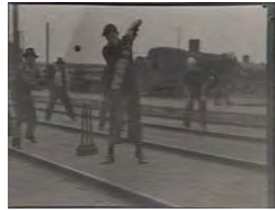
Figure 3.65: Cricket played between the lines, presumably at the Carriageworks or the Alexandria Goods Yard south of the Locomotive Workshops. Source: ML Picman Citation no.: NCY40/289 Frame no.: Home and Away - 17156.
