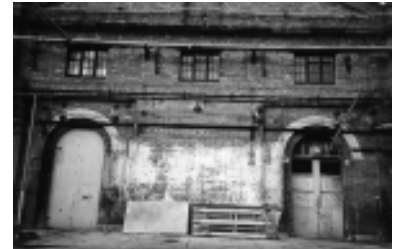
Figure 3.87: 1998 photograph of the northern external wall of Bay 21 showing the doors fitted to either side of the original opening which had been filled in. Source: Jean Rice.
