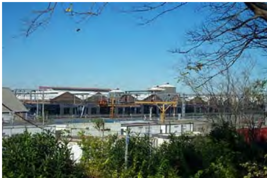
Figure 5.2: Views of the former Locomotive Workshops from the CME's garden today. A visual connection between both sites is important to maintain at some level, to remind and inform of the historical link between the two sides. This view shows the repetitive facade and the three higher towers added to accommodate industrial processes in the building. Photo: Jean Rice 2002.
