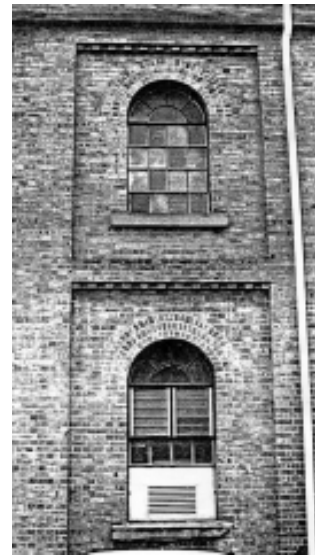
Figure 3.172: (above) Honeysuckle Point Workshops, NSW, exterior view. Note the double columns and lattice girders, identical to Eveleigh. The roof trusses are timber. Doring, Honeysuckle.
