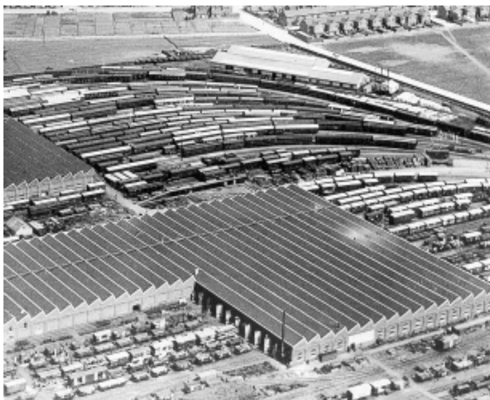
Figure 3.165: Aerial view of the original wagon shops at Swindon taken in 1922. This was the largest concentrated repair unit in the United Kingdom but its activities were transferred to the Locomotive Works in 1967. Note the fan of rails which is similar to, but larger than, the fan to the east of the Paint Shop at the Eveleigh Carriage Workshops and it appears not to feed into a shed. Source: 'An Illustrated History of British Railways' Workshops' p 145.
