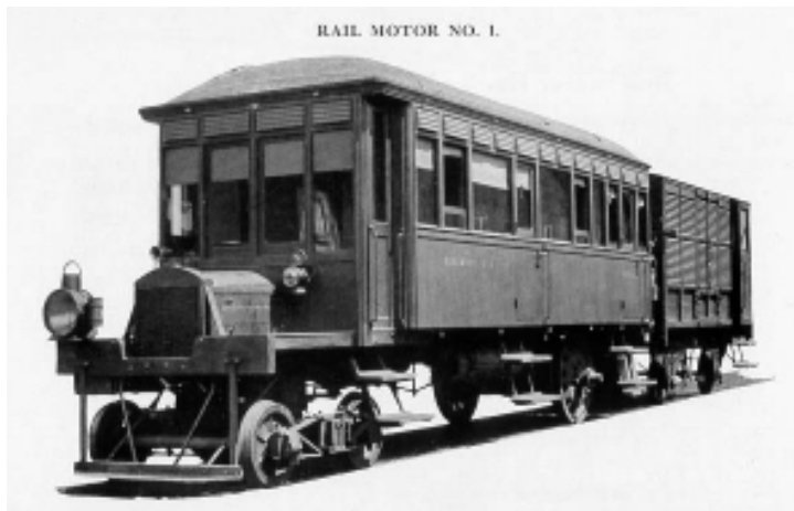
Figure 3.109: New South Wales first Rail Motor which was converted from a motor lorry at the Eveleigh Carriageworks in 1919. Source: "The Railways of New South Wales 1855-1955", p171.
