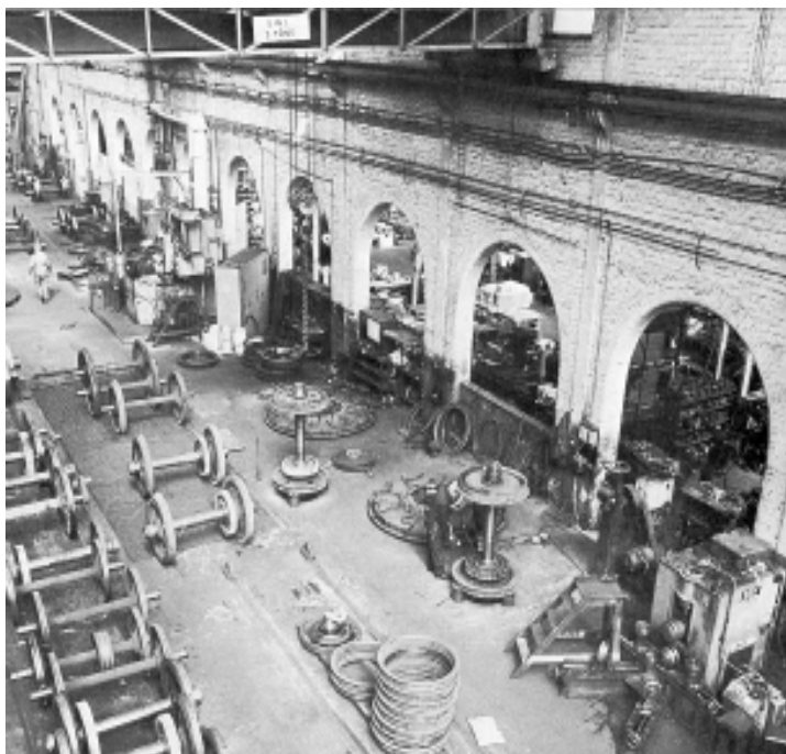
Figure 3.162: St. Rollox (Glasgow) Railway Workshops. Source: 'Railway Architecture' p 170.
