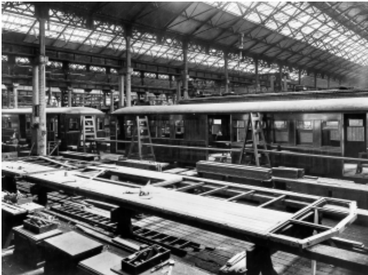
Figure 3.77: Interior of Bay 17, showing construction of timber carriage floor of the 42' rail motors. Undated but probably in the mid 1920s. Source: SRAO
