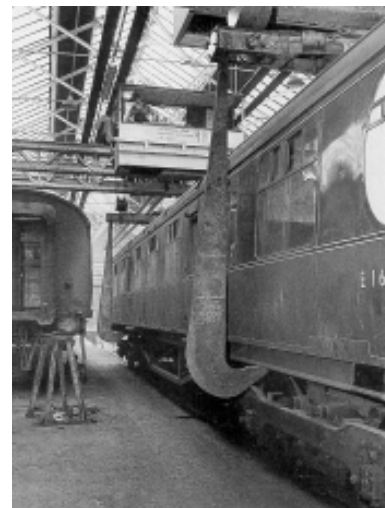
Figure 3.70 : Carriage Lifting at York Carriage Works, England, undated. Carriages were lifted in a similar way at the Carriage Lifting Area at Eveleigh. Source: 'An Illustrated History of British Railways' Workshops' p 127.
