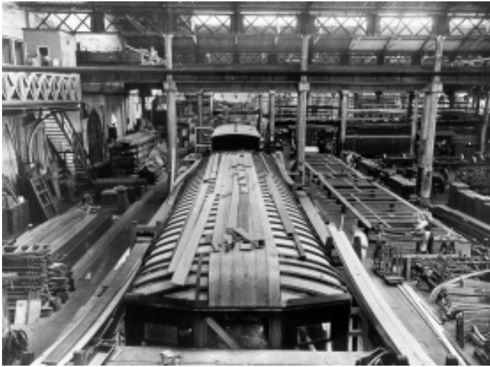
Figure 3.76 : Interior of Bay 17, where the original traverser had been located, showing the building of the 42' rail motors. Undated but probably in the mid 1920s. Source: SRAO
