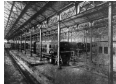
Figure 3.92: Interior of the Paint Shop in 1891, facing west. The large south-facing skylights appear to have been the only light source at the time. Source: ML, The Illustrated Sydney News , 18th July 1891
