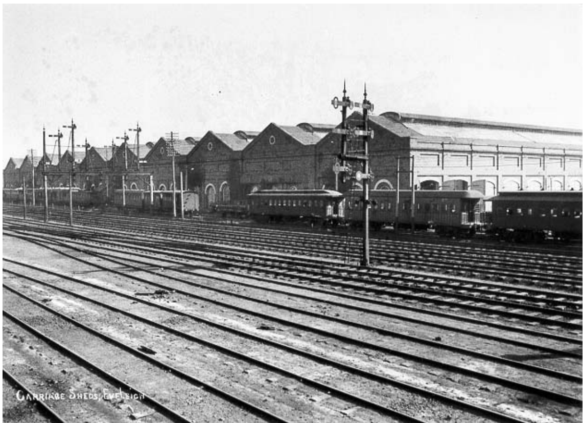
Figure 4.0: View of the Carriage and Wagon Workshops in 1910. Source: Mitchell Library Videodisk GPO I Still No. 12020.
