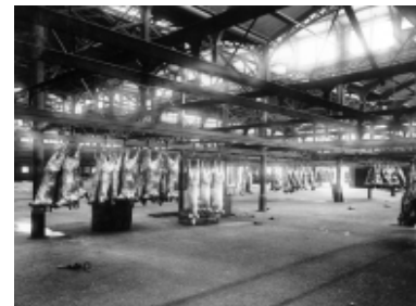
Figure 3.141: Meat Markets, Darling Harbour. Interior view. The photograph shows round cast iron columns, wrought iron trusses and iron roofs. Source: Sharkey Collection, PWD.
