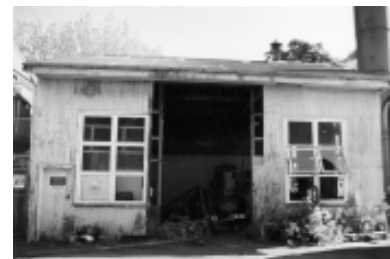
Figure 3.47: Compressor House built c.1913. Source: Otto Cserhalmi, 1998.
