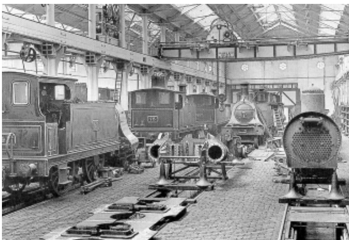
Figure 3.138: Interior of the Erecting Shop at Bow Locomotive Works in 1898. The 'Craven' crane is similar to those in the Eveleigh Carriage Works main building. In railway workshops, bay width, and therefore roof span, was limited by the need to support the crane. Source: 'An Illustrated History of British Railways' Workshops' p 31.
