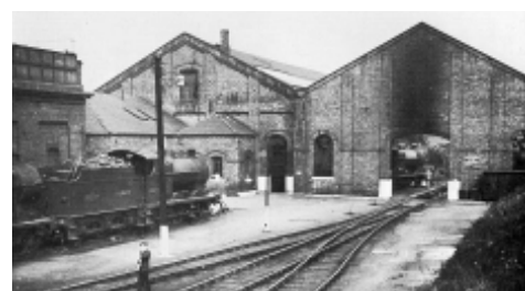
Figure 3.167: Running Sheds at Hasland, near Chesterfield, built for the Midland Railway. This two-bay example is similar to the sheds at the Redfern Railway Yards (refer Section 3.1.2) and is of an earlier date than the Eveleigh Carriage Workshops. Source: 'Railway Architecture' p 169.
