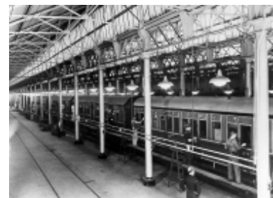
Figure 3.93 : Undated photograph of the interior of the Paint Shop, facing east. The Bay in the foreground is probably Bay 6a which did not have a pit. Note the electric lights which had probably been installed in the 1920s. Source: SRAO
