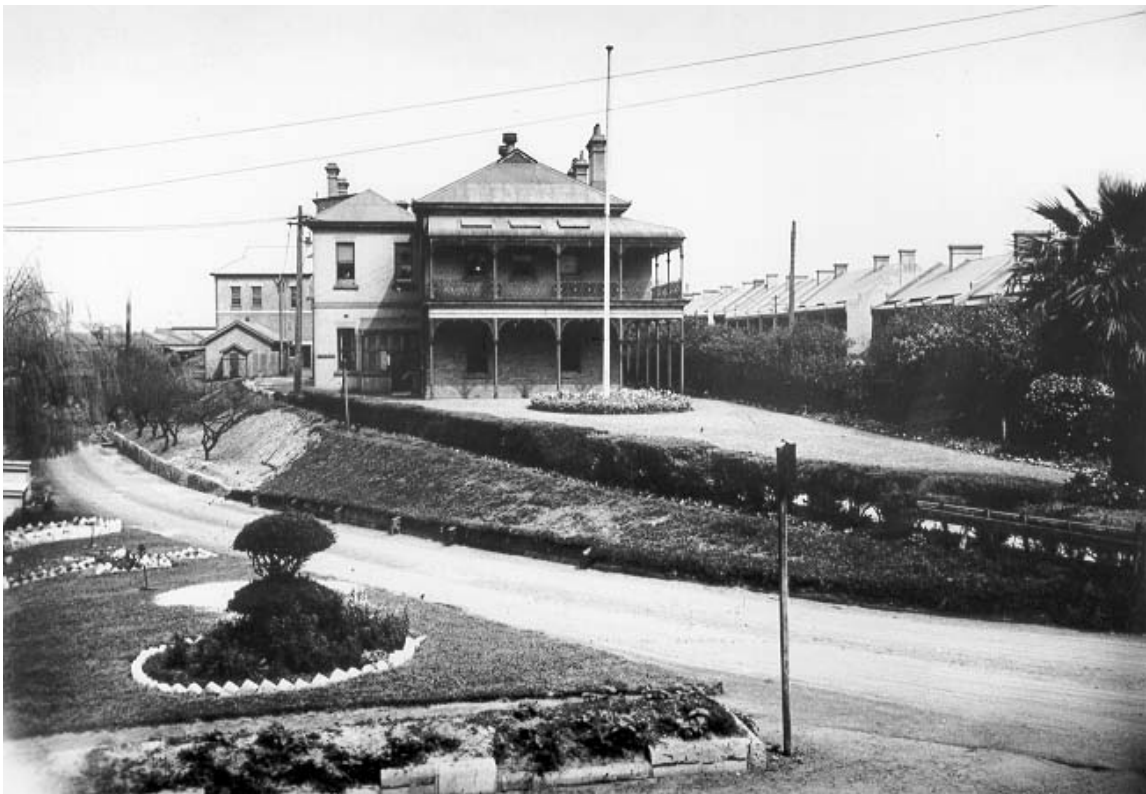
Figure 3.27: Chief Mechanical Engineer's Offices, Wilson Street. Undated (post 1900) view from North East. Source: SRAO.
