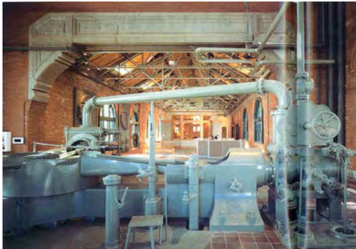
FORMER SEWAGE WORKS, BOSTON MASSACHUSETTS
