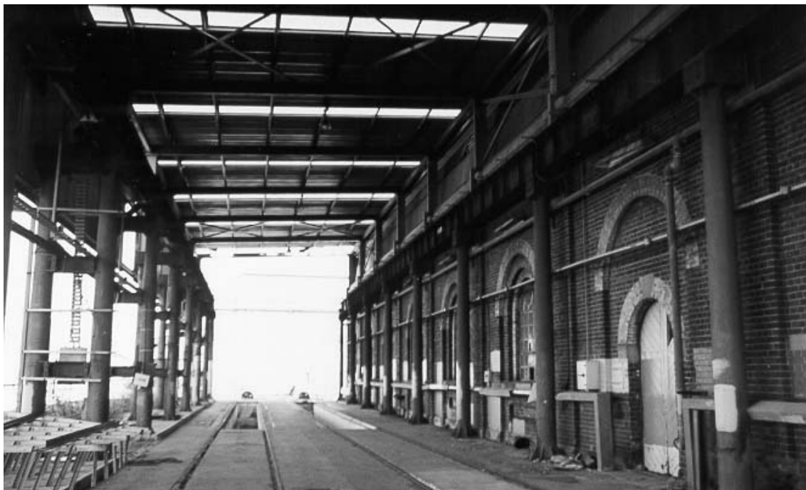
Figure 6.0 : The south wall of the Paint shop. Here the carriages were lifted off their bogies and onto workshop bogies. The worn bogies were then moved to the bogie repair shop and the carriage to the carriage repair shop. When the repairs were complete each carriage was reunited with its bogie before return to service.
