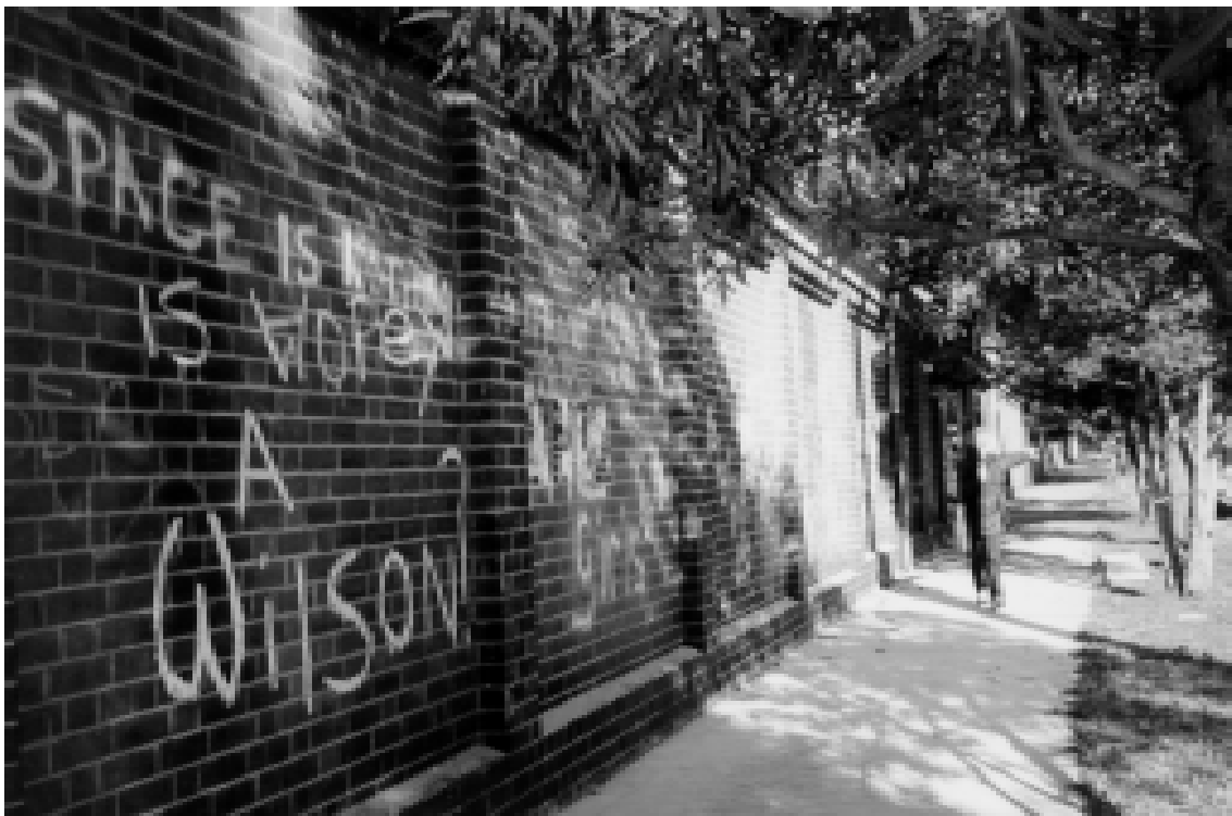
Figure 6.0: The Wilson street side of the retaining wall. On the other side is the Blacksmiths' Workshop. Photo: OC+P.
