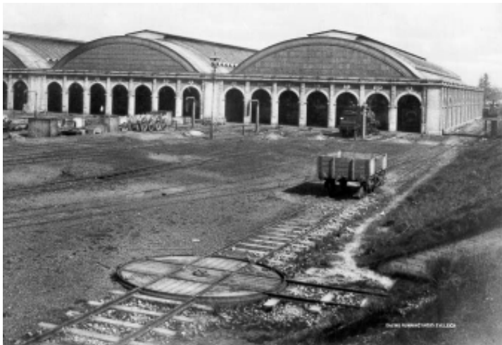
Figure 3.23: Photograph of the wagon turntable located at the southern (Locomotive Works) side of the access tunnel under the main lines with the Running Shed (now demolished) in the background. c. 1884. Source: ML Videodisc GPO 1.
