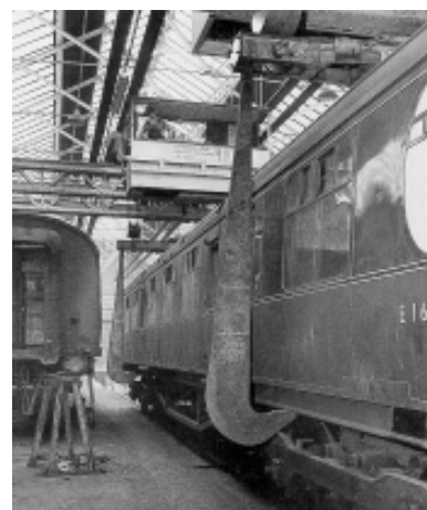
Figure 3.166: Lifting carriages at York Carriage Works - the general practice for lifting coaches on and off their bogies by means of two cranes. A similar technique would have been used in the Carriage Lifting area adjacent to the Paint Shop at Eveleigh Carriage Workshops.
