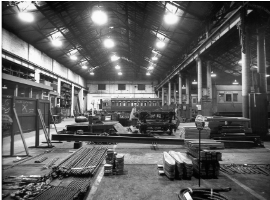
Figure 3.81: Interior of Bay 21 entitled 'Production Control Shop'. Probably 1943. Source: SRAO
