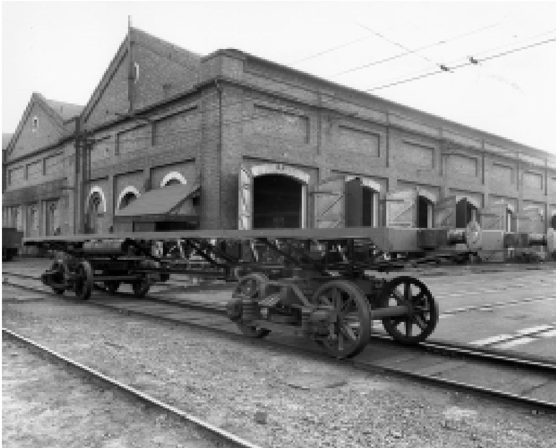
Figure 5.1: View of the Carriage Workshops taken from the southeast. Undated. Source: SRAO.
