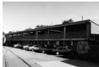
Figure 3.56: Fire Protection and Drug Analysis Building 1998. Source: Otto Cserhamli.
