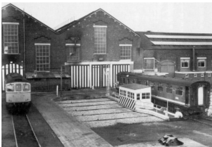
Figure 3.160: Eastleigh Carriage and Wagon Works was built in 1891 by the London and South Western Railway Company on a 54 acre site. The works constructed new carriages and repaired carriages, wagons and containers. By 1968, the repair work had been transferred to the Locomotive Works and the site was sold. Note the traverser, very similar to those at the Eveleigh Carriageworks, transporting a carriage in the foreground. Source: 'An Illustrated History of British Railways' Workshops' p 141.
