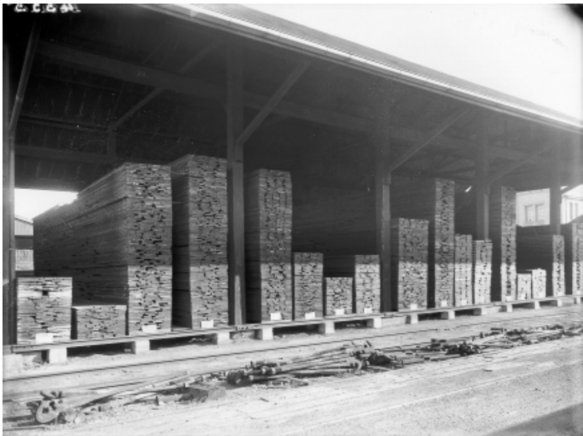
Figure 3.71: View of the Timber Shed extension 1953. In this building and the main Timber Shed were stored the sections of timber which would be used in carriage repair, overhaul and construction work. During World War II, the Annual Reports note that timber was difficult to obtain and that several carriages were therefore built from timber which was already in stock. This building is there as of 2002. Source: SRAO
