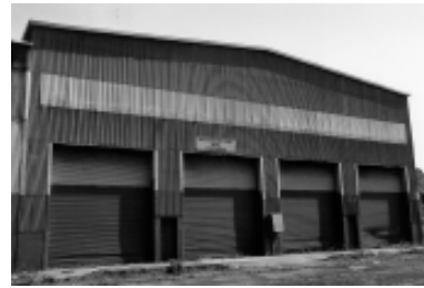
Figure 3.54: Boilermakers' Shop, 1998. Source: Otto Cserhamli.
