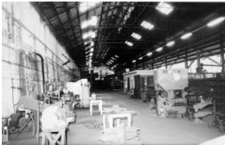
Figure 3.99 The Blacksmiths' Shop in 1986. The two heavy pedestal grinders are against the Wilson Street retaining wall with the K15 metal shears and punch and metal rack to the south of the centre line of the building
