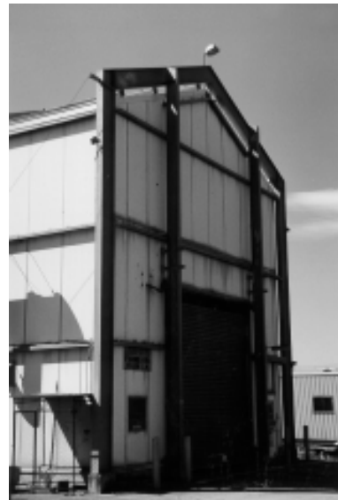
Figure 3.55: Asbestos Removal Shed, 1998. Source: Otto Cserhamli.
