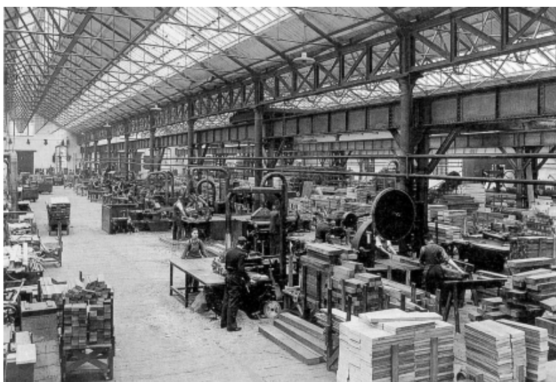
Figure 3.157: The sawmill of the above works in 1922. The arrangement is very similar to Eveleigh Carriage Workshops with cast iron columns separating the bays. Unlike at Eveleigh, a separate structure appears to support the crane girders in the adjacent bay. Source: 'An Illustrated History of British Railways' Workshops' p 109.
