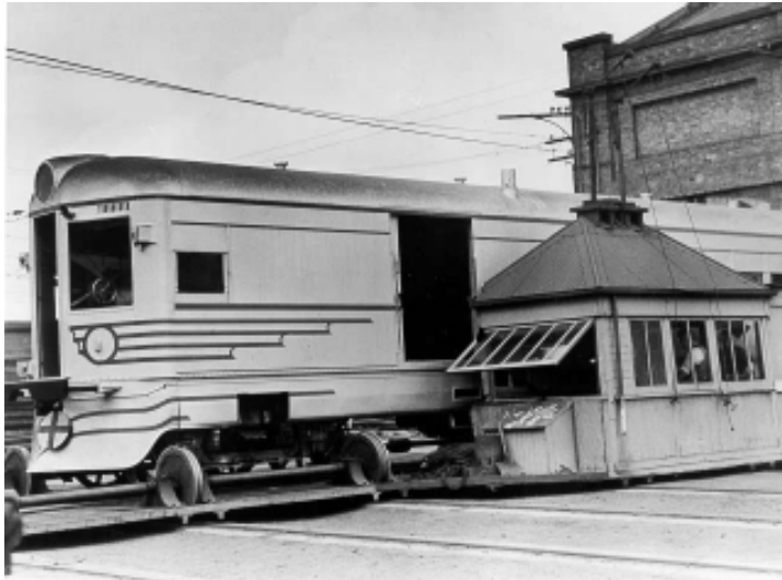
Figure 3.108: A 400 class Rail Motor on Traverser No. 1 at the Eveleigh Carriageworks c.1937. This traverser was originally located inside the main workshop but was moved outside between the Carriage Workshop and the Paint Shop in 1901. It ran on 600v DC power with two overhead wires. This traverser was replaced by a more modern one that was relocated from Yennora in 1971. Source: SRAO.
