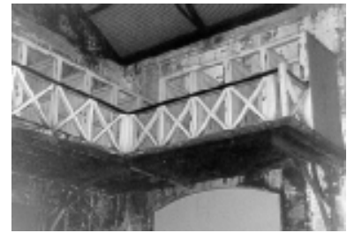
Figure 3.86: 1998 photograph showing the elevated toilet block in the south western corner of Bay 25. Source: Otto Cserhalmi.
