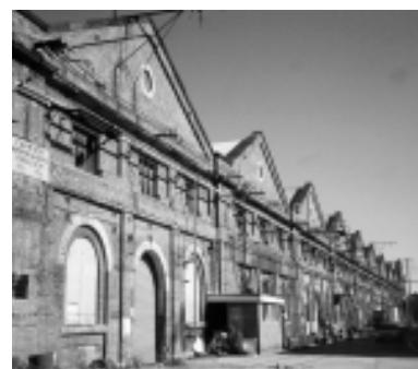
Figure 3.139: Northern elevation of the Eveleigh Carriage Workshops, 1998. The building is typical of Victorian industrial buildings and demonstrates masonry exteriors designed to conform to nineteenth century taste. Source: Jean Rice
