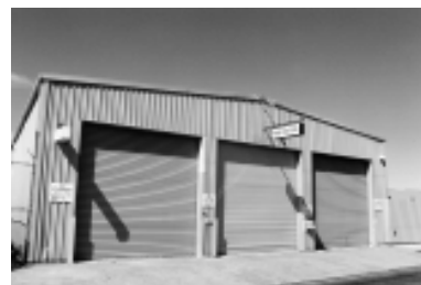
Figure 3.57: Fire Protection Brigade Shed 1998. Source: Otto Cserhamli.
