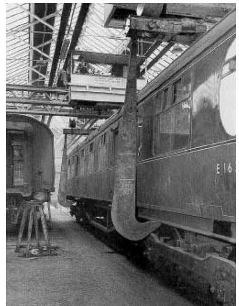
Figure 3.100: Lifting carriages at York Carriage Works - the general practice for lifting coaches on and off their bogies by means of two cranes. A similar technique would have been used in the Carriage Lifting area adjacent to the Paint Shop at Eveleigh Carriage Workshops. Source: Larkin 1992: 127.
