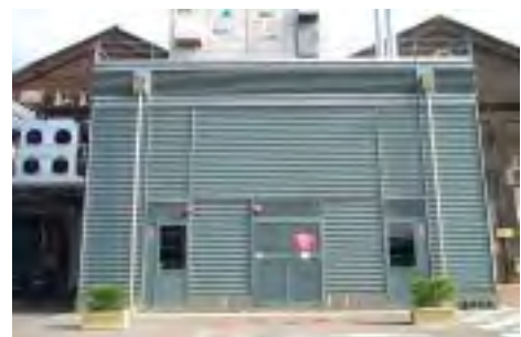
Figure 3.28: Modern industrial detailing to the new annex added in 1996. Source: OC+P
