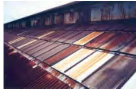
Figure 7.18: Original skylight configuration, Bay 15 west. Source: Otto Cserhalmi, 1996.
