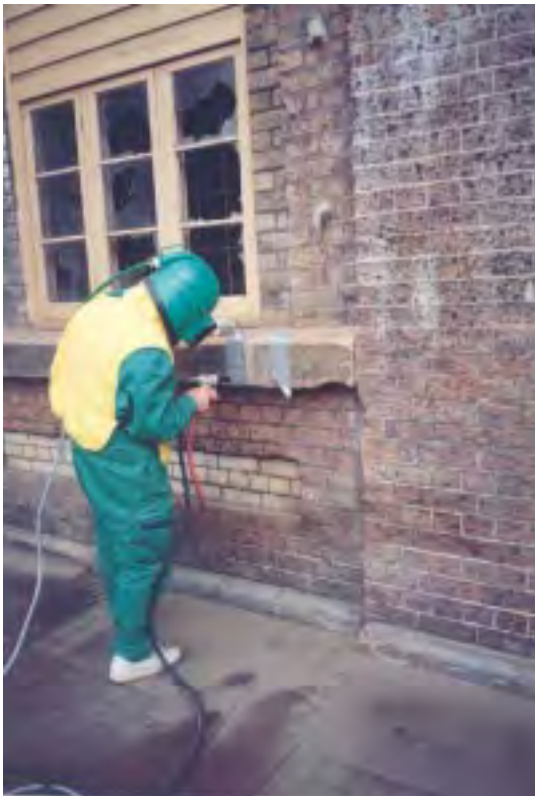
Figure 7.21: Testing a sandstone cleaning method on a small square of sandstone sill. Source: Otto Cserhalmi 1996.
