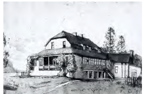
Figure 3.9: Calder House in 1921. Etching by Sydney Ure Smith. It is not known whether these illustrations are of the same building or not. It is conceivable that the building could have been altered from the vernacular form to the upper Victorian form but this would mean the date of this etching is wrong. Source: ML PXN 670, DG* D43
