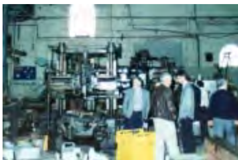
Figure 3.26: Machinery moved and stored in Bay 3 while the building was in use by Paddy's Markets. Source: David Sheedy.
