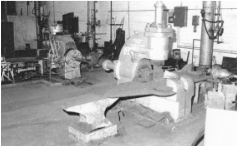
Figure 4.60: Bay 4 North. The Fielding & Platt hydraulic spring buckling press was used to assemble leaf springs. Photo by D. Godden 1985.
