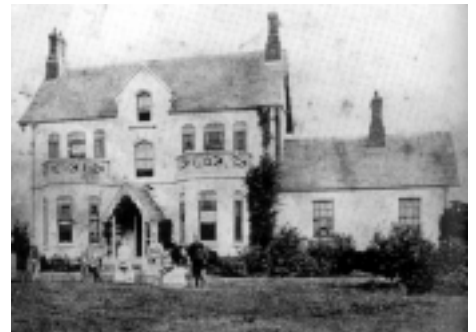
Figure 3.8: Calder House at the Redfern Station end of Wilson Street. It housed the managers of the Eveleigh Railway workshops and burnt down in 1921. Note that the etching below is identified as Calder House also although it appears to be a different building. Source: Sharpe 1999: 78.
