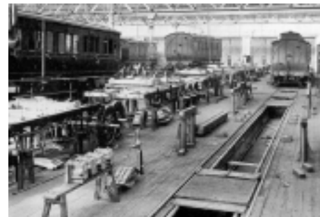
Figure 3.90: Early photograph of the Carriage Lifting Shop in Derby Carriage Works at Litchurch Lane. The works was built in 1876 for the Midland Railway on a site of 128 acres. They were designed to handle carriage construction from raw materials to finished stock. By 1948, the site was the principal carriage and wagon works of the railway and employed over 5000 staff. In 1962, new wagon work ceased, repairs were drastically cut and the works was adapted to cater solely for carriage work which was still continuing at the site in 1992. Source: Larkin 1992: 109.
