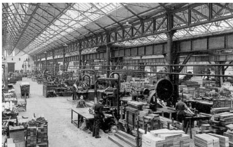
Figure 3.91: The sawmill of the above works in 1922. The building arrangement is very similar to Eveleigh Locomotive Workshops with cast iron columns separating the bays. Unlike at Eveleigh, a separate structure appears to support the crane girders in the adjacent bay. The machines must be operated by electric motors or hydraulics as no line shafting is visible. Source: Larkin 1992: 109.
