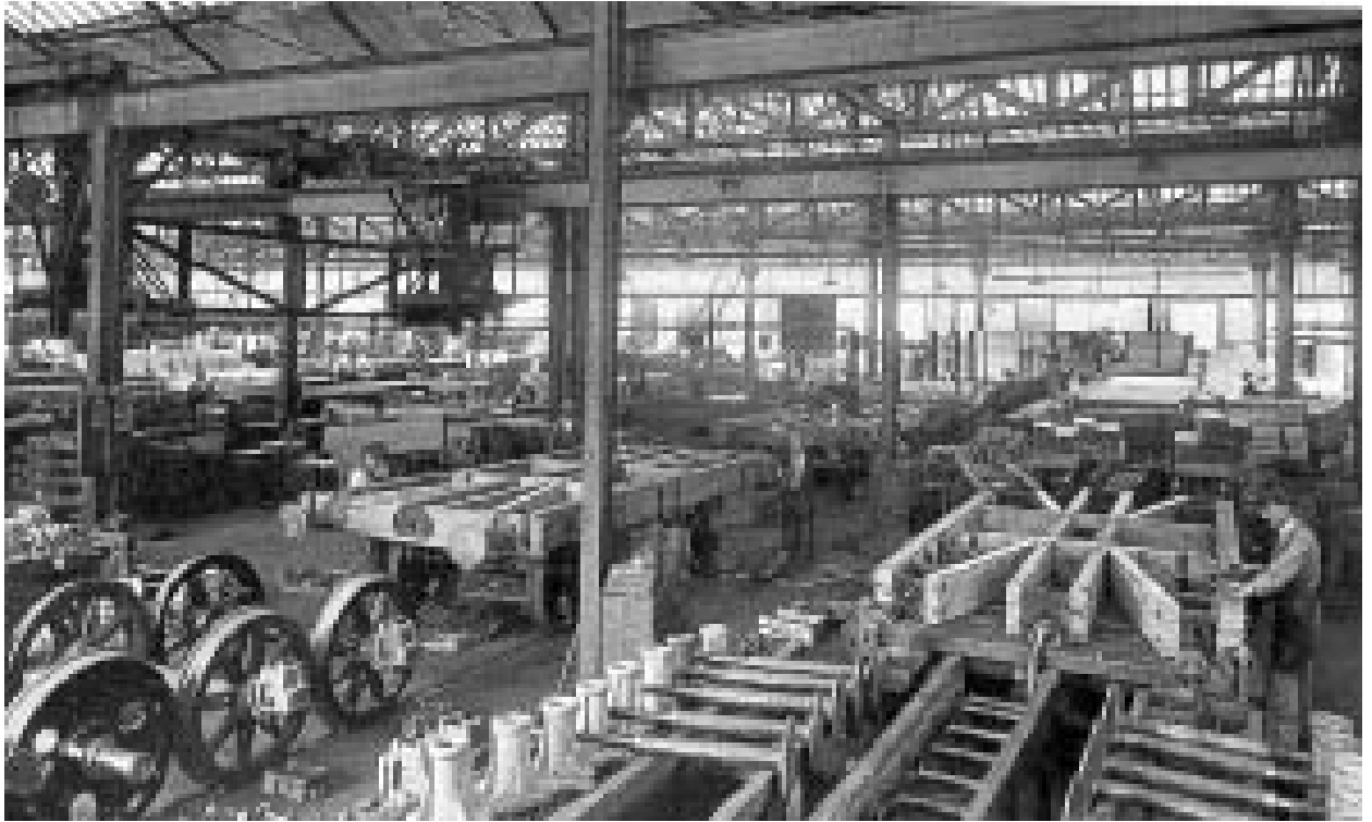
Figure 3.92: Building wooden wagons of 12 ton capacity at Derby Litchurch Lane Carriage and Wagon Works during the period 1924-1930. Source: Larkin 1992: 138.
