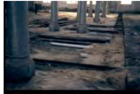
Figure 4.3: Rails revealed during construction work in 1996. Photo: OC+P 1996.
