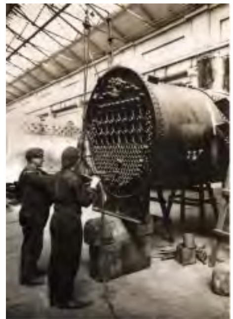
Figure 3.55: Bay 4a looking south-west showing rolling of tubes with pneumatic tube expanders to D53 class boiler. SRAO ELW 601/47.
