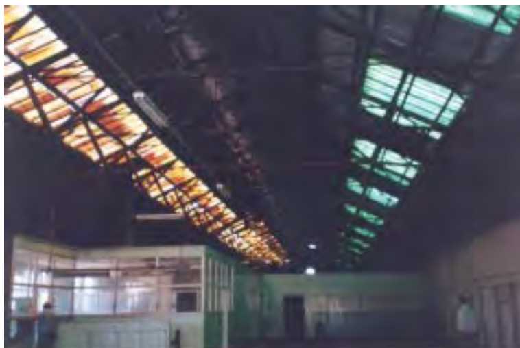
Figure 7.19: Original configuration of glazing in Bay 15 west (old Bay 14). Photo: Jean Rice 1995.
