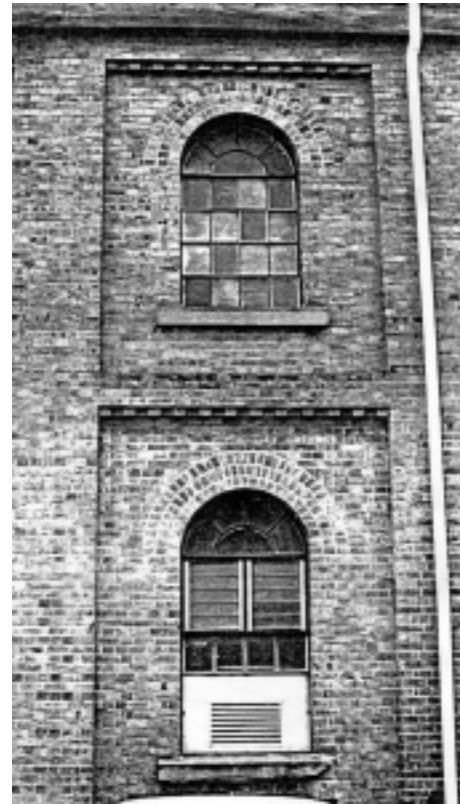
Figure 3.105: (Above) Honeysuckle Point. Detail of former Locomotive Boiler Shop, showing brickwork detailing, stone sills and cast iron windows, Doring, Honeysuckle.
