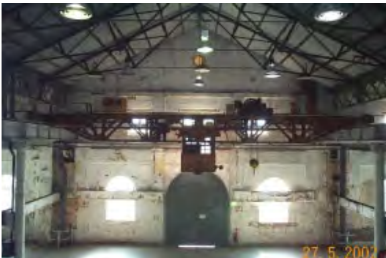
Figure 7.23: Bay 12 looking north. The crane is supported by the crane rails on either side. Original light fittings are still in situ on either side of the third row from the front (see Policy 5.11.2). Photo: Istvan Czehmester 2002.
