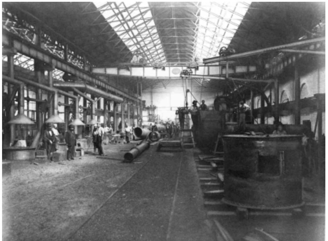
Figure 3.32: Interior view looking south along Bay 3, prior to the wall on the right being demolished. Note the wall engine at centre back. The flues correspond with the flues on the original plan. Source: ML GPO Video Disk 06681 Sh 976, 1884.
