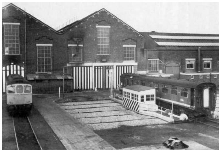
Figure 3.94: Eastleigh Carriage and Wagon Works was built in 1891 by the London and South Western Railway Company on a 54 acre site. The works constructed new carriages and containers and repaired carriages, wagons and containers. By 1968, the repair work had been transferred to the Locomotive Works and the site was sold. Note the traverser, very similar to those at the Eveleigh Railyards, transporting a carriage in the foreground. Source: Larkin 1992: 141.
