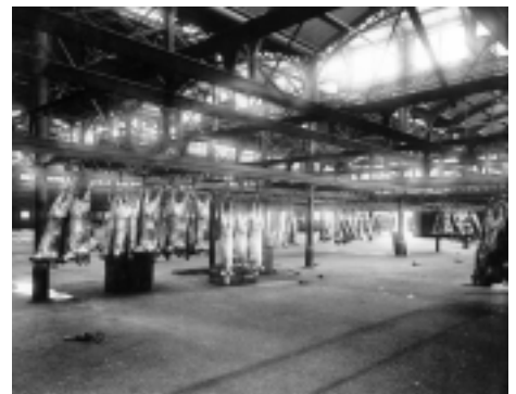
Figure 3.74: Meat Markets, Darling Harbour. Interior view. The photograph shows round cast iron columns, wrought iron trusses and iron roofs, Sharkey Collection, PWD.
