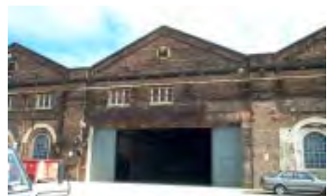
Figure 3.29: The traverser opening in these days has been utilised as a vehicle entry. The detail of the doors is derived from the original design. Source: OC+P
