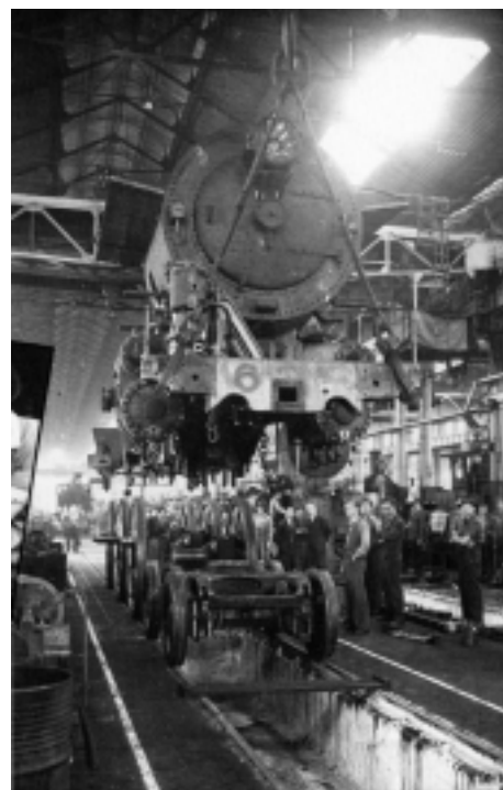
Figure 3.20: A C38 being lowered to the wheels in the Large Erecting Shop at Eveleigh, west of the Locomotive Workshops. This building remains in SRA ownership and use. Source: Burke 1988:191.
