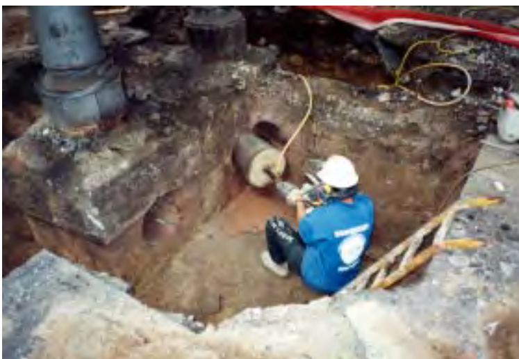
Figure 4.80: Bay 1. Boring under foundations to check the efficacy of the original downpipe system
