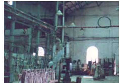
Figure 4.52: Racks of tools adjacent to forges in Bay 2 north. Photo by OC+P 1998.
