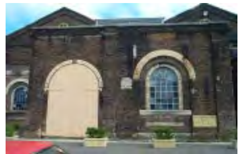
Figure 4.20: Annex 13, South Wall. Photo: Jean Rice 2002.
