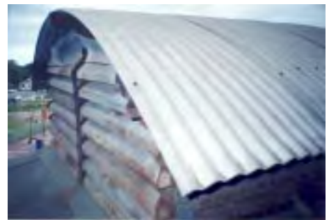
Figure 4.13: Detail of end of roof monitor showing metal louvres. These may have been removed in 1996. Photo: OC+P 1995.
