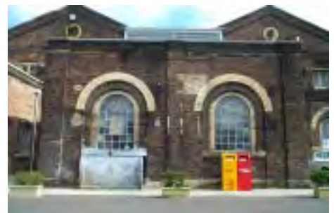
Figure 4.19: Annex 12, South Wall. Photo: Jean Rice 2002.
