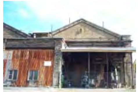
Figure 4.18: Annexes 1 & 2, South Wall. Photo: Jean Rice 2002.
