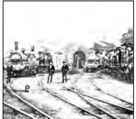
Figure 3.16: Redfern Terminal Engine Sheds, early 1870s. The design of these sheds is typical for the type and they are similar to English models. Source: Burk, 1988: 10.
