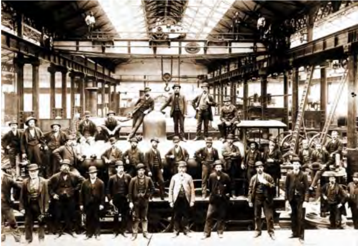
Figure 3.53: Erecting Shop in the Locomotive Workshops, c1886 with locomotive in foreground under repair. The locomotive is over one of the pits that ran across the bay. The photo shows the rope drive 1884 Craven crane and the workmen dressed up especially for the photograph. Bay 6 looking north from central road with traverser bay on l.h.s. (Bay 7). SRAO ELW 601/17
