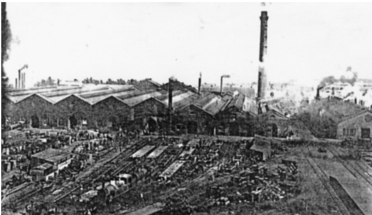
Figure 3.104: Newport Railway Workshops, Melbourne. Historical view of half of the complex which is repeated to the left of this photo. Note the configuration of the building in bays and how the fan of rail lines serve each bay, Doring, Newport.
