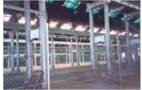
Figure 4.12: Column grid, Bay 6 looking north-west. This area has since been enclosed with construction. Photo: Jean Rice, 1995.
