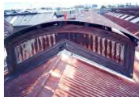
Figure 4.32: Detail of end of roof lantern showing corrugated sheeting and moulded timber detailing. These may have been removed in 1996. Photo: OC+P, 1995.
