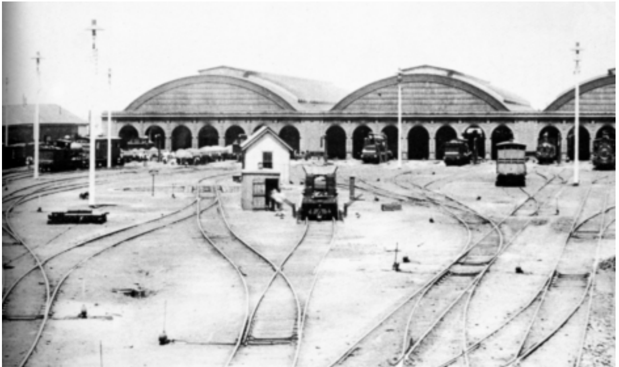
Figure 3.21: Eveleigh Engine Running Sheds, 1887. Exterior view showing Cowdery's segmental arched roofs each covering seven "roads". The last bay was demolished in 1960. Source: Burke, 1988: 142-143.
