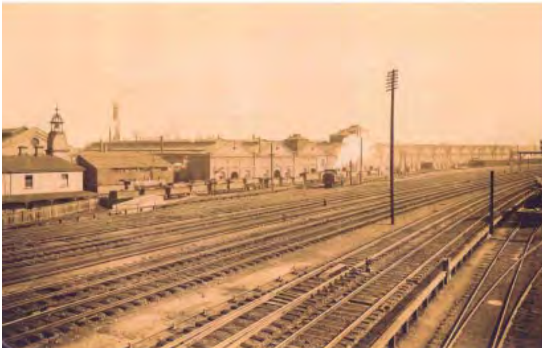
Figure 3.37: View from Redfern overbridge. Bay 3 has a high level window. Note the chimney stack behind the workshops at the left of the photo, the additional tower, which now total three, Bay 4a has been enclosed, Bay 7 still has the traverser opening and the Spring Shop is to the north of the Workshops. SRAO ELW 601/41
