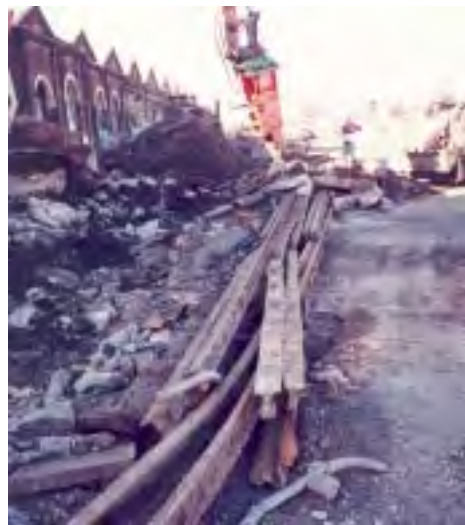
Figure 3.24: Removal of rail on the southern side of the building. Source: OC+P
