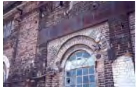
Figure 4.6: Detail, south wall Bay 14 (old Bay 13), showing early infill to the traverser opening removed during 1996. Photo: Jean Rice 1995.
