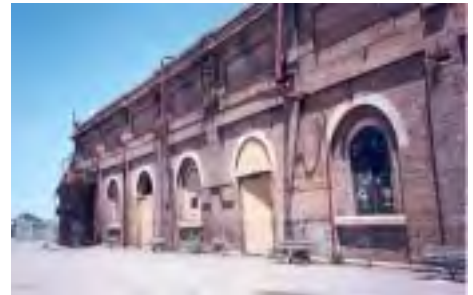
Figure 4.5: East wall, Rows 1 - 6, prior to conservation work. Photo: Jean Rice 1995.
