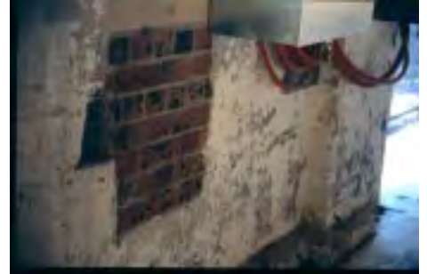
Figure 7.14: Test panel of cleaning techniques showing original bricks under layers of intrusive paint. It is recommended that maintenance test panels are not located in prominent areas (see Policy 5.2.2).
