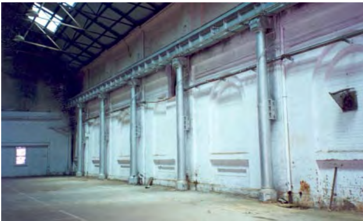
Figure 4.1: Bay 5 (Old Bay 4a), west wall looking south. This was originally an external wall with the column and crane rail added when the bay was enclosed. Photo: Jean Rice 1995.
