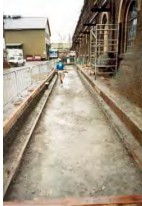
Fig7.28: The external traverser track on the western side of the Locomotive Workshop. These tracks are still there, but now covered over. Photo: OC+P 1996.
