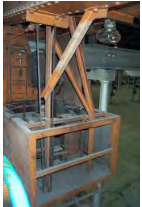
Figure 7.19: Crane operators' cabin, Bay 13 (old Bay 12). Photo: Istvan Czehmester, 2002.
