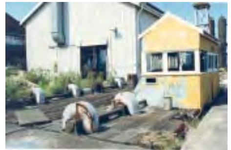
Figure 4.79: The traverser in its bed next to the Spring Shop. The southern wall of the Locomotive Workshops can be seen in the left of the photograph. Both the traverser and Spring Shop have been removed. Photo: ATP Archives.
