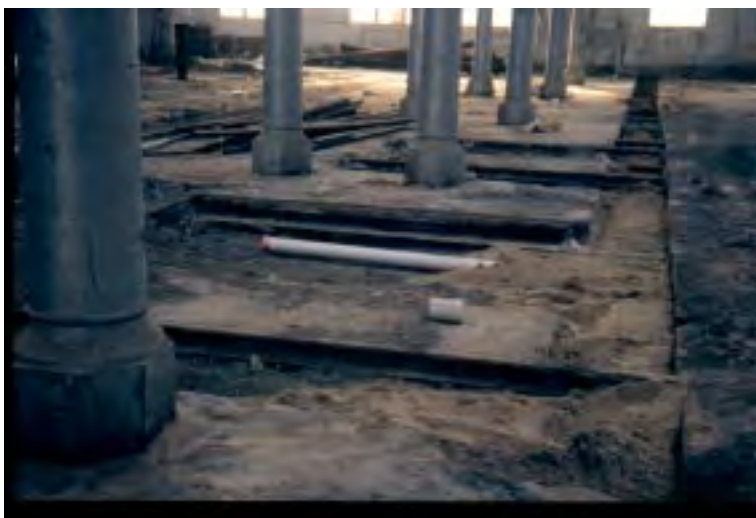
Figure 7.24: Bay 10 - 14 (old Bays 9 - 13) Engines were moved along the length of Bay 8 (old Bay 7) or Bay 15 (old Bay 14) by the traverser and then across Bays 10 - 14 along the rails exposed in this photo, to where they would be worked on. Photo: Otto Cserhalmi, 1996.
